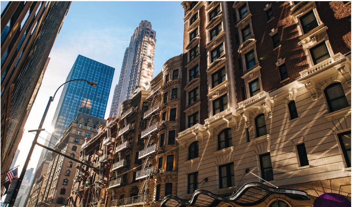
Figure 4-45: Facade, New York City
