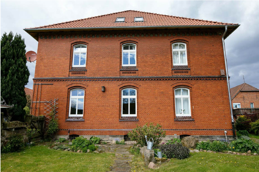
Figure 6-5: Tilting the camera enables you to fit the entire building into the frame but makes it look as if it is tipping backward.
